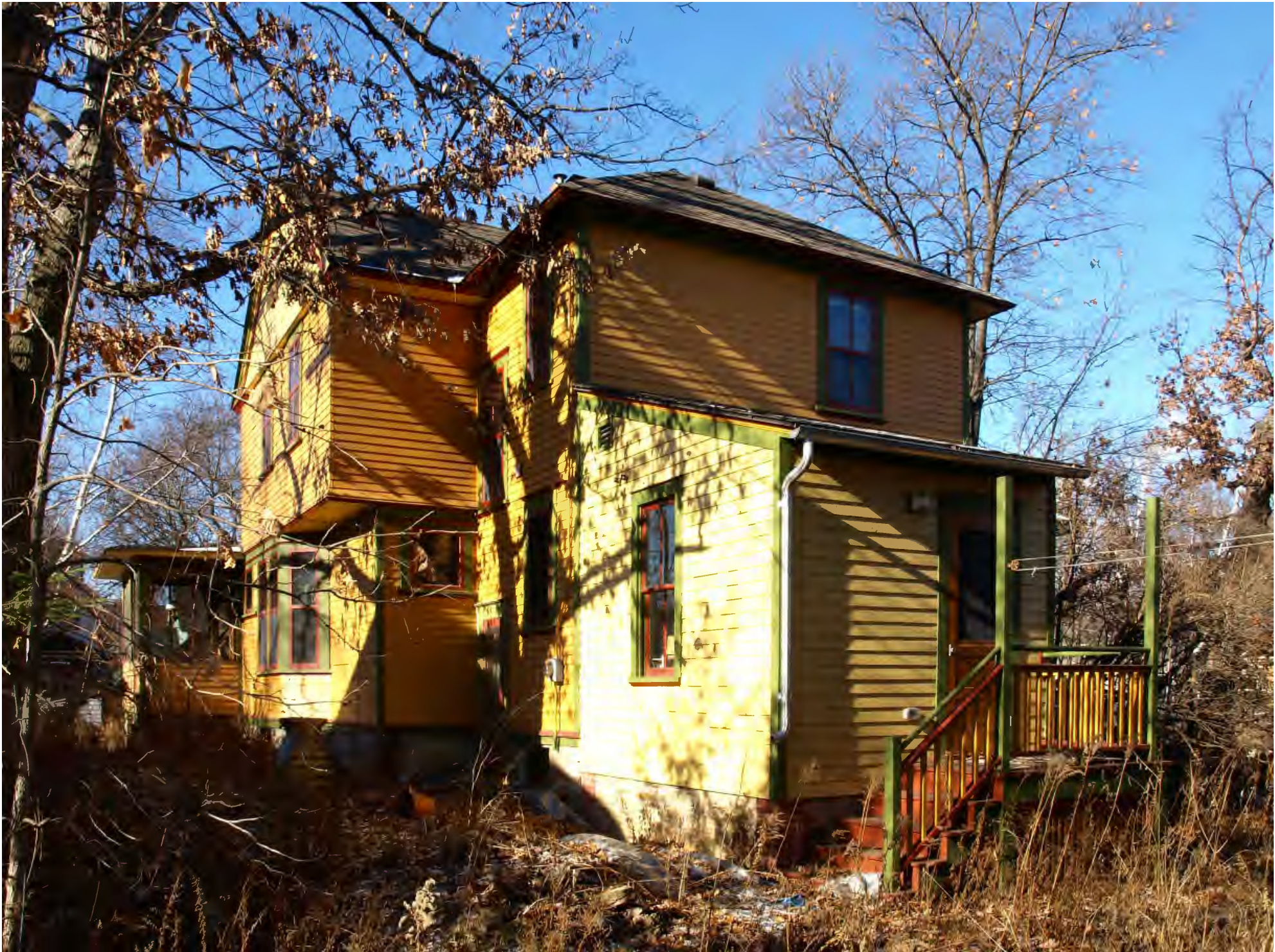
Dwight and Clara Watson House_0003 house viewed from southeast standing b barn, south and east elevations, camera facing northwest
