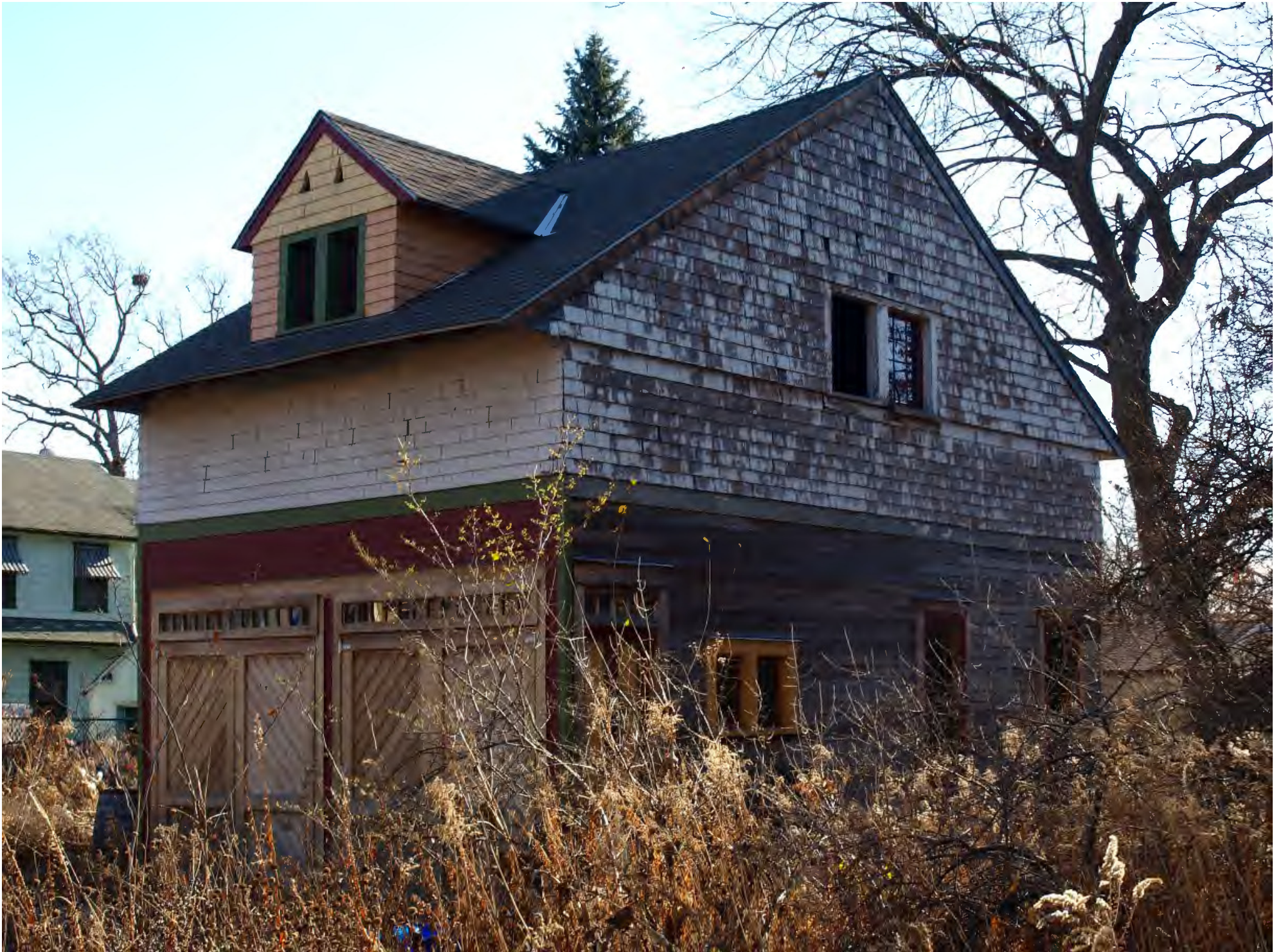
Dwight and Clara Watson House_0010 barn viewed from northwest, north and west elevations, camera facing southeast
