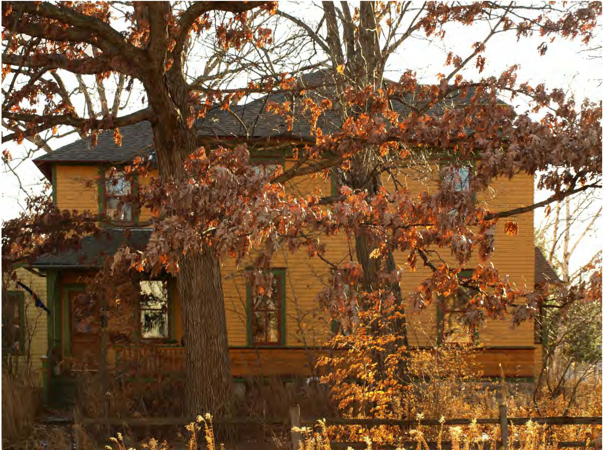
Dwight and Clara Watson House_0004 house viewed from north, north elevation, camera facing south
